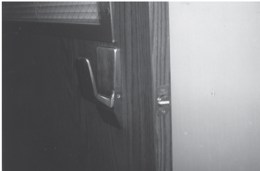
Figure 6-5. Lever Latch. The lever latch works similar to a door knob but the lever has advantages because persons with limited ability to grip a doorknob or operate at thumb latch. This photo shows a door to a patient room in a hospital. ( Photo by Robert Reid, 2004 )
