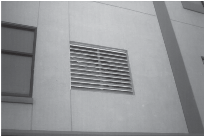
Figure 5-9. Ventilation opening for an office building. While many building ventilation openings are for the roof, or below ground with a grille, some facilities continue to have ventilation openings on the side of the building. (Photo by Robert Reid, 204)
