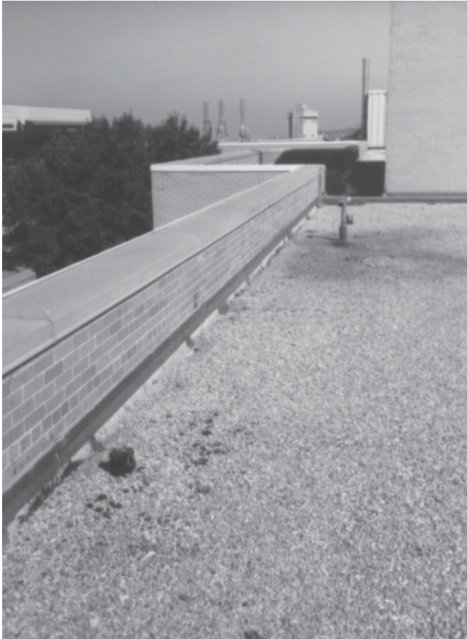
Figure 4-1. Parapet wall. The problem with this type of wall is that the wall can catch explosive devices that will fall off of a sloped roof. (Photo by Robert Reid, 2004)
