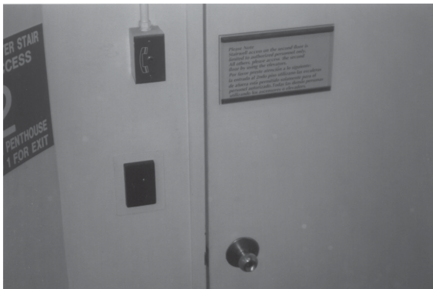
Figure 8-3. Proximity Reader. This photo shows a typical proximity reader installed in a stairwell of a hospital. The secured area is the maternity ward. (Photo by Robert Reid, 2004)
