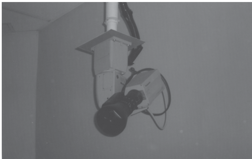
Figure 11-3. Indoor pan, tilt and zoom camera. (Photo by Robert Reid, 2004).
