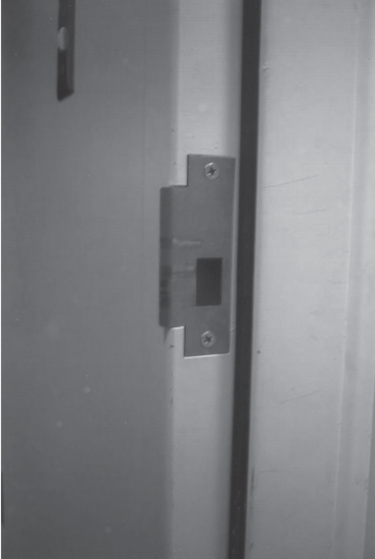
Figure 6-1. Strike and Strike Pocket. The edge of the jamb where the door closes is called the “strike.” The metal hole in the door that catches the latch is called the “strike pocket.” (Photo by Robert Reid, 2004)
