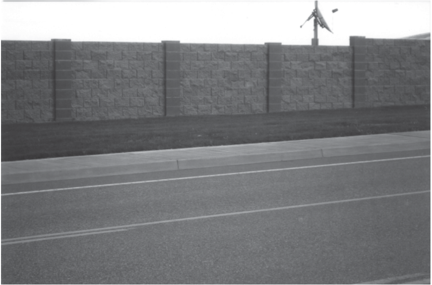
Figure 3-9. Block walls provide good perimeter security, but they are expensive. (Photo by Robert Reid, 2004)
