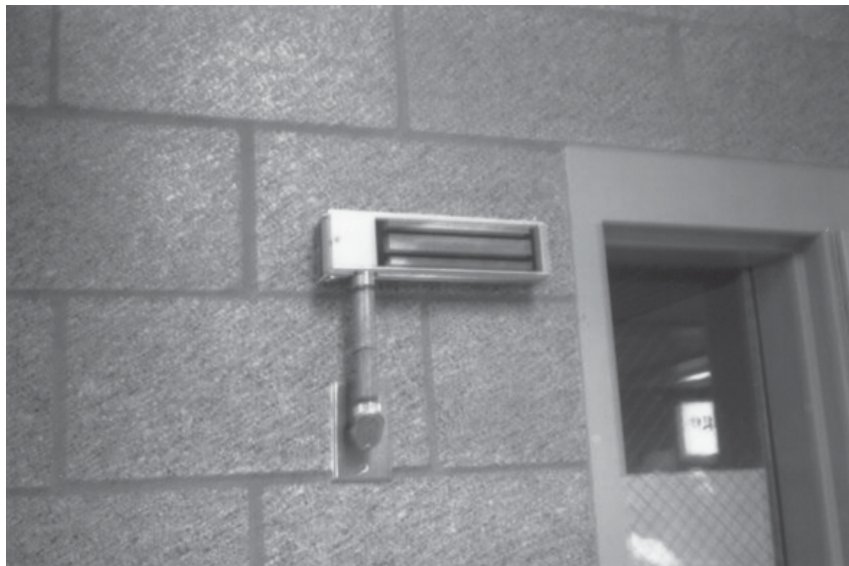
Figure 7-1. Electromagnetic Lock. This electromagnetic lock is being used in a school to hold doors open. The device can also be mounted to hold the door closed. ( Photo by Robert Reid, 2004 )
