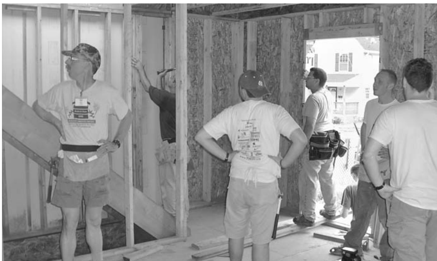
FIGURES 3.15 AND 3.16. The Carrier House project by the Hartford Area Habitat for Humanity features OVE using engineered lumber.
