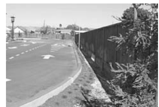
FIGURE 3.3. The bioswale system at Nuevo Amenecer helps improve the quality of water draining off the site.
