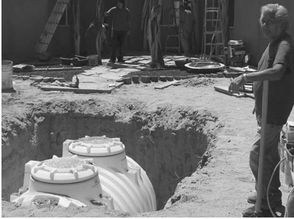
The home's roof design collects rainwater through inverted shed design, and it is then stored in a buried water tank.
