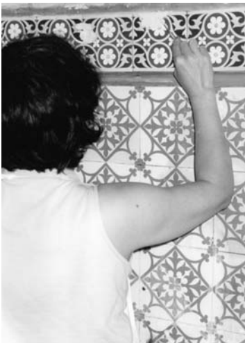
Figure 7.15 Polyester resin filler being applied to damage.
