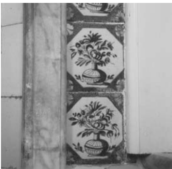
Figure 5.28 Full restoration on delft tiles.
