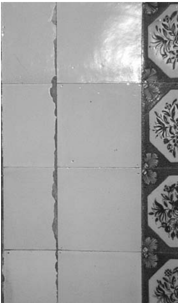
Figure 5.2 Typical damage to the glazed edges of delft tiles.
