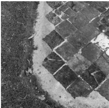
Figure 7.18 Lime mortar 'buffer' zone.
