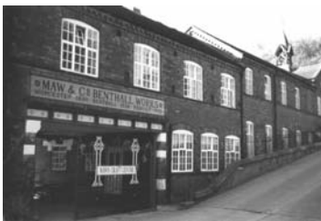
Figure 2.18 The old Maw & Co. tile factory at Jackfield, Shropshire.
