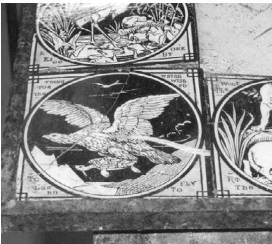
Figure 5.24 Fracturing caused by corrosion expansion.
