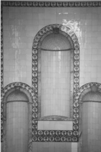
Figure 3.8 The niches, Carshalton Water Tower, Surrey.
