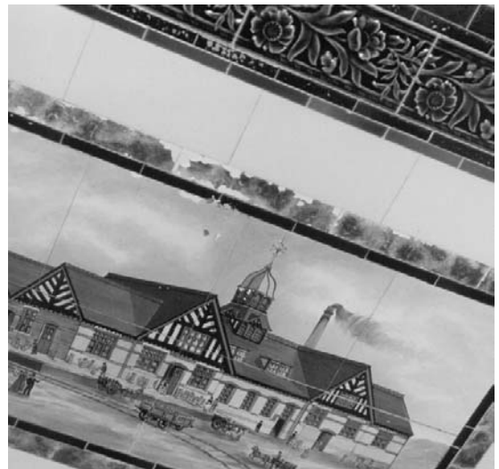
Figure 5.23 Spontaneous shedding of glaze due to tensile pressure.
