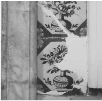
Figure 5.27 Plaster infill in eighteenth century tiles.
