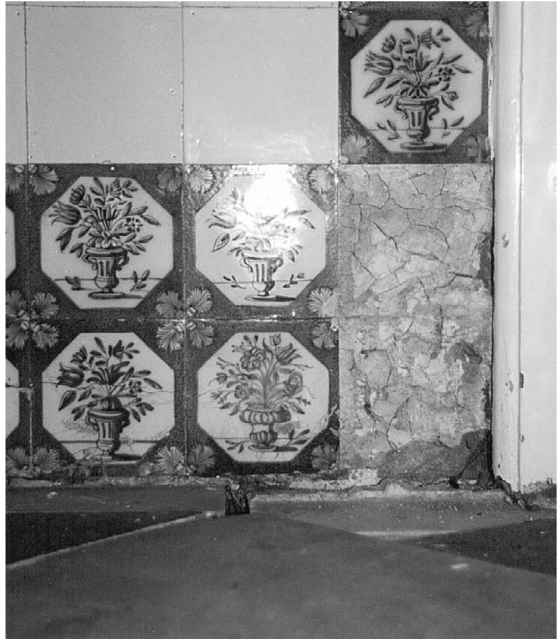
Figure 3.11 Eighteenth century mortar substrate, Carshalton Water Tower, Surrey.
