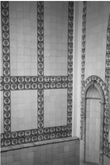
Figure 3.7 Carshalton Water Tower, Surrey.
