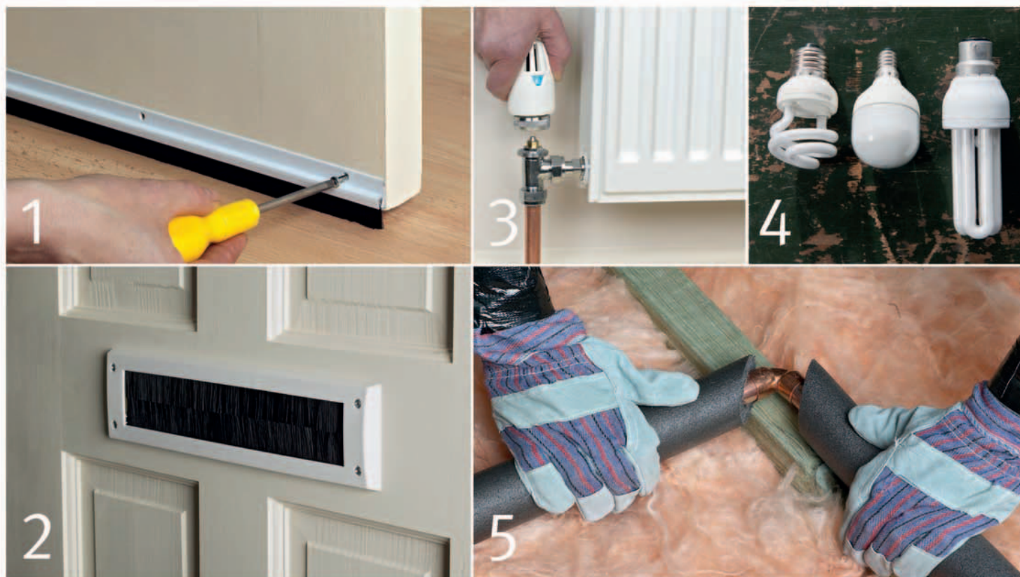
1. Add door sweeps to all external doors to keep your home warm. 2. Draft-proof a letterbox with brush strips. 3. Thermostatic radiator valves allow you to heat rooms to different temperatures. 4. Low-energy light bulbs are available in options to suit all fixtures. 5. Insulate pipes in a cold attic to reduce heat loss.
