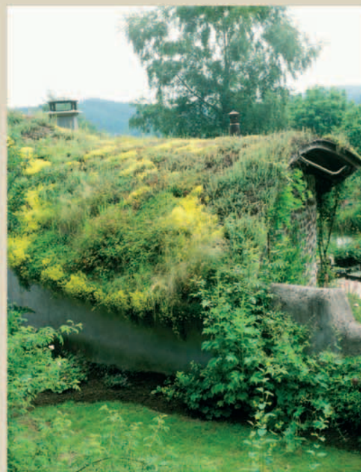
A sedum roof can be installed on a flat or sloping roof, but the incline should ideally be less than 25°. You'll need access to the roof from time to time to weed it and water if necessary in dry spells.
