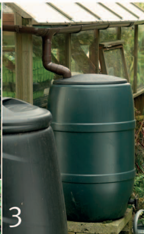
1. Pump water directly from a stream for a domestic water supply if you don't have a well or spring. 2. Battery-powered pump draws water from the stream to irrigate the greenhouse. 3. Rain barrels are the simplest way to collect rainwater from sheds and greenhouse roofs for your garden.
