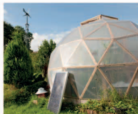
The shape of a geodesic dome prevents warm air pockets from forming, making it ideal for growing plants under cover.
