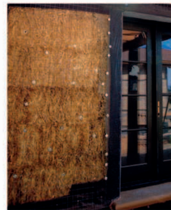
A wooden frame built with bale-sized spaces between the uprights is the perfect support.
