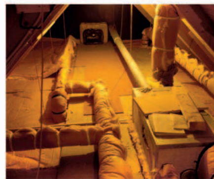
A heat recovery unit installed in an attic. The pipes running to and from the unit are insulated to prevent heat loss.
