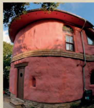
Lime plaster can be colored with pigments or painted after it dries.
