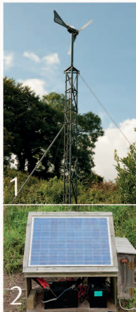
1. Our grid-linked wind turbine allows us to sell any excess electricity we create back to the power company. 2. Energy created by these solar PV panels is stored in deep-cycle batteries for such things as pumping water from our spring.
