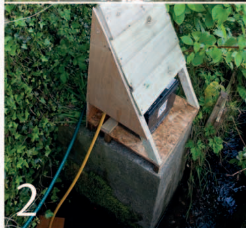
1. Pump water directly from a stream for a domestic water supply if you don't have a well or spring. 2. Battery-powered pump draws water from the stream to irrigate the greenhouse. 3. Rain barrels are the simplest way to collect rainwater from sheds and greenhouse roofs for your garden.
