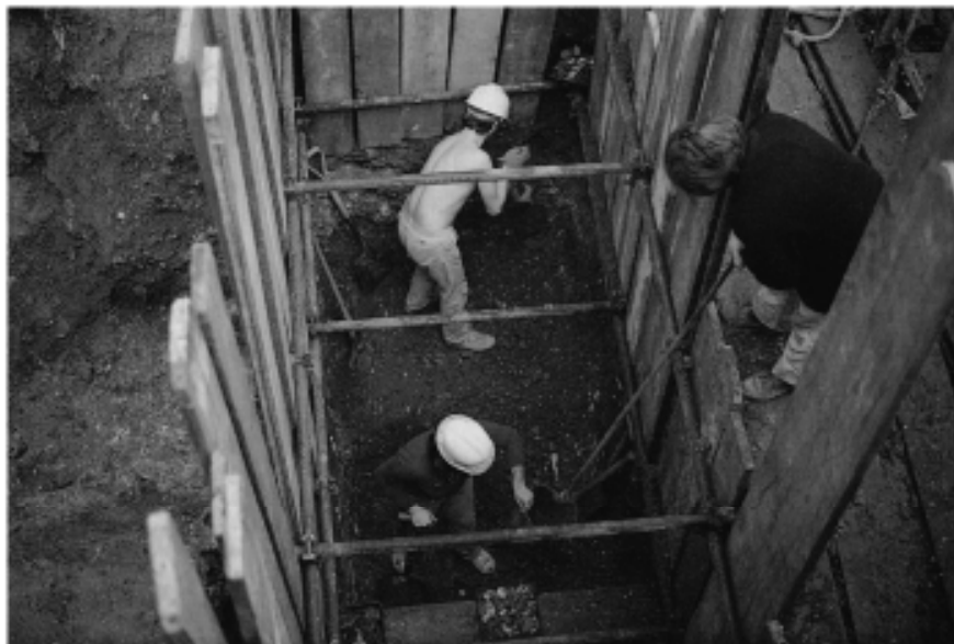
Figure 5.2 Site safety: shoring of a narrow trench.
