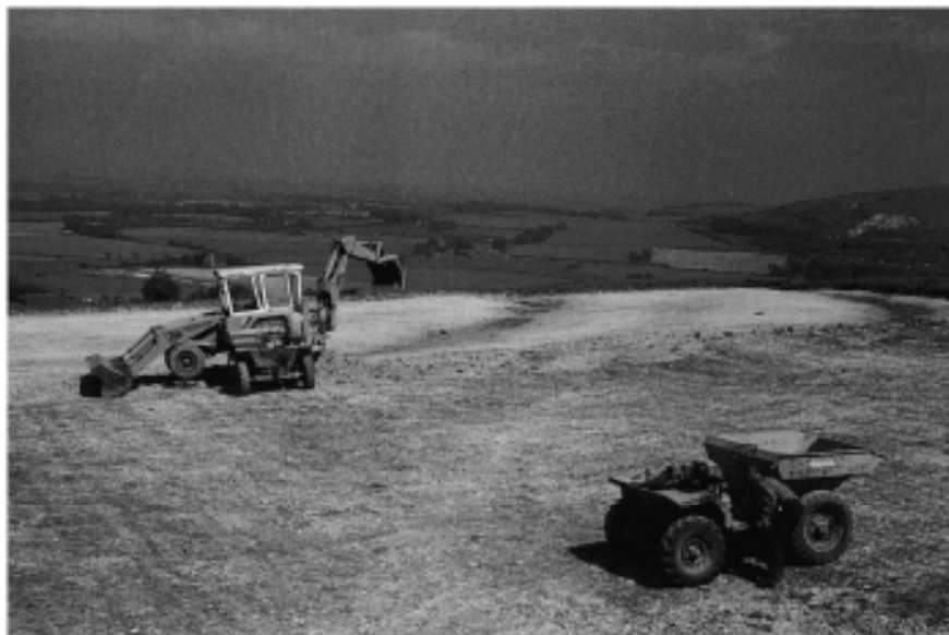
Figure 5.13 Coarse excavation: digging with a JCB 3c.
