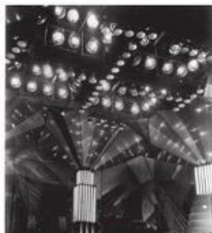
FIGURE 1.3 Early tungsten units in use on the set of Broadway . The dome-shaped units were called “rifles” for their ability to project light at a distance. The open-face units were called “Solar Spots”. Films were “slow” back then (meaning they needed large amounts of light to get a good exposure). Lenses were also slow; the result was that sets had to be lit to a very high lighting level. (Photo courtesy of Mole-Richardson Co.)
