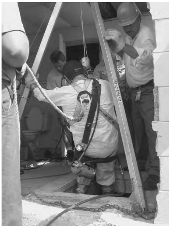
Figure 1.2 Lowering a well-protected city worker into a sewage-holding tank in search of human remains.
