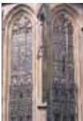
Great Tower windows
