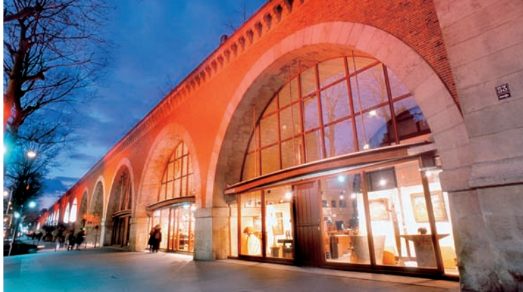
Shops in the Viaduc des Arts.
