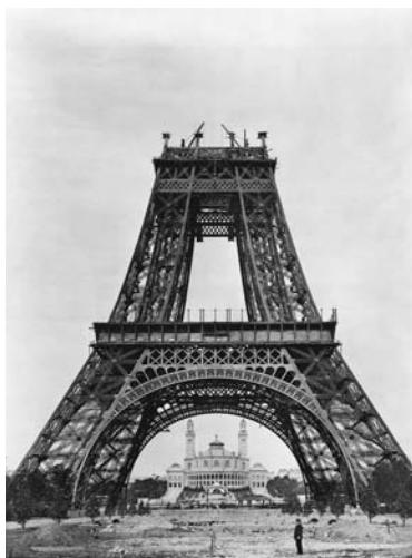
Tour Eiffel under construction.
