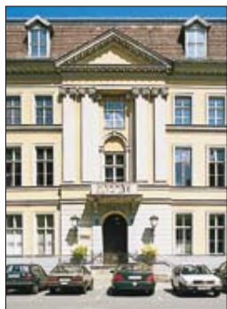
Facade of the twice-restored Palais Podewils
