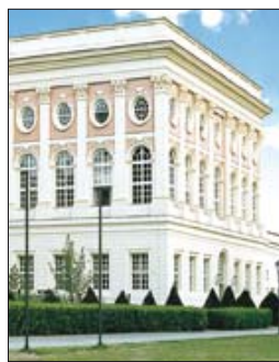
Elegant façade of the Communs, the servants' quarters
