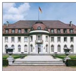
The Villa Borsig façade viewed from the garden
