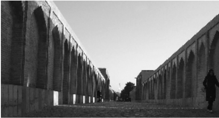
The upper level of the Khajou Bridge.
