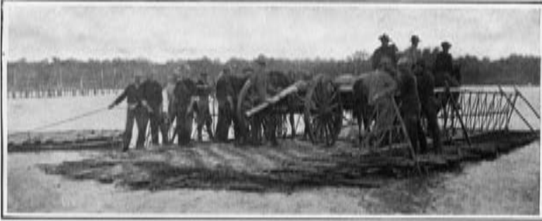
A Bamboo Ferry hastily built by United States Engineers—Ferrying a Piece of Artillery across the River near San Fabian
