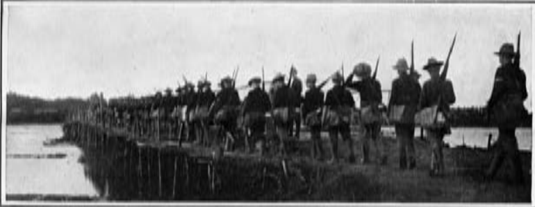
Bamboo Bridge built by United States Engineers across the River near San Fabian for Troops and Wagons to Cross
