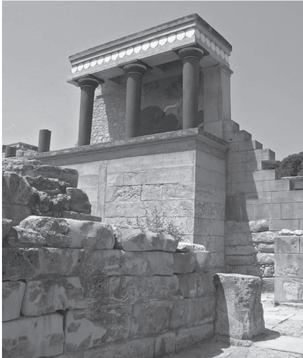
7.6. North Entrance Passage, Palace at Knossos. Photo by author.
