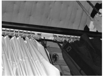
Figure 19.106 Day/night curtain on grid pipe system rail.
