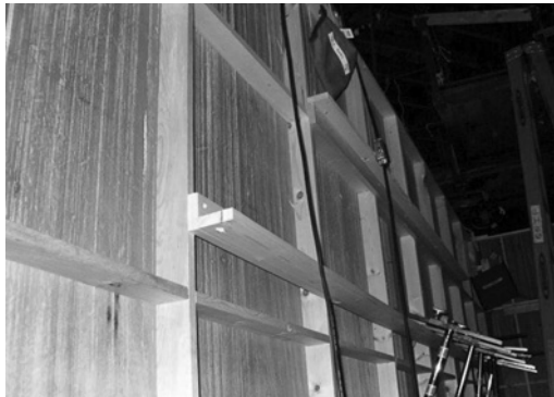
Figure 19.118 Hog trough horizontal brace strongback.
