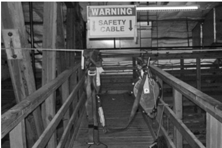
Figure 19.91 Safety harness on steel cable (fall protection).
