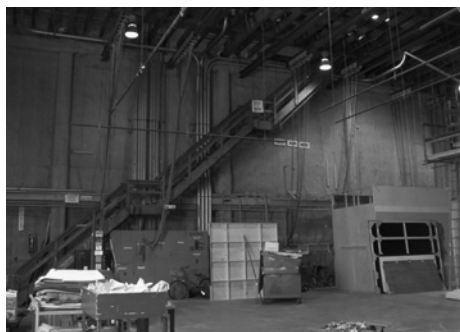
Figure 19.79 The stairs up.
