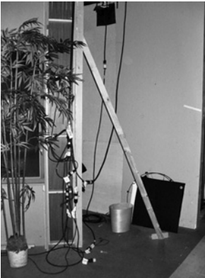
Figure 19.117 Stage wall. Notice the blocks of wood nailed to brace/ground.
