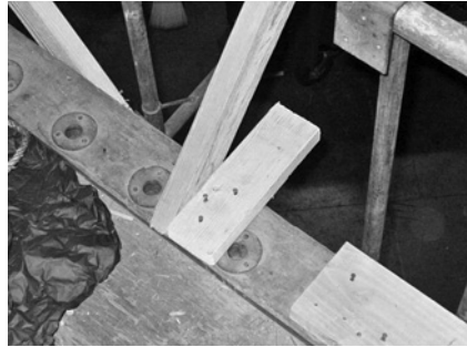
Figure 19.96 2 × 4 braces to prevent swinging (a.k.a. the kicker).
