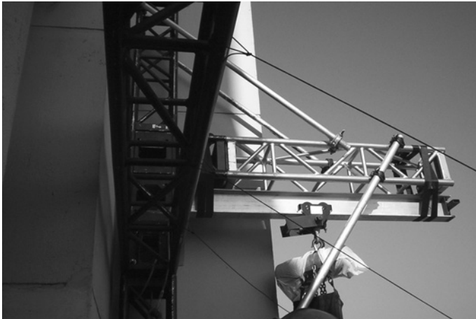
Figure 19.141 Brace/kicker to sliding chain motor.
