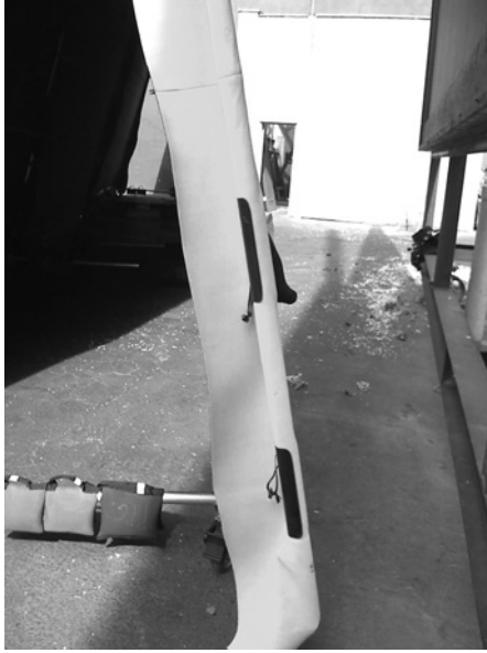
Figure 19.7 Green screen held on with speed clips.
