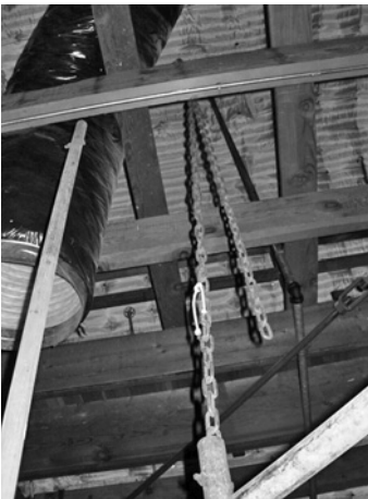
Figure 19.94 Hung from the perms by chain.
