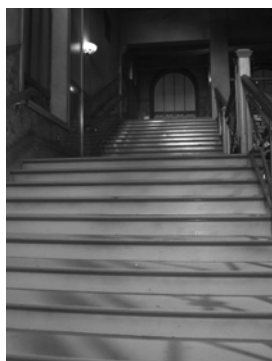
Figure 19.109 Stairway to “nowhere.”
