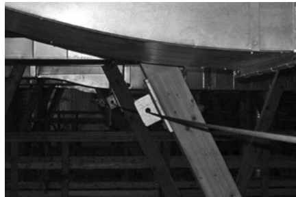
Figure 19.92 Cable attached to the perms.
