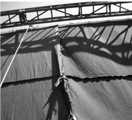
Figure 19.13 Grip clips on ribbon to prevent tears in the blacks.
