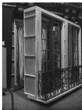
Figure 19.111 Rolling plugs (moving set walls).
