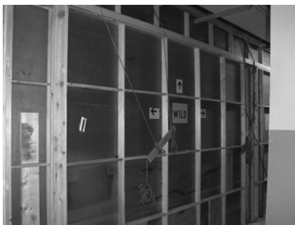
Figure 19.128 Wild Wall (easy removal); a.k.a. flyaway wall.
