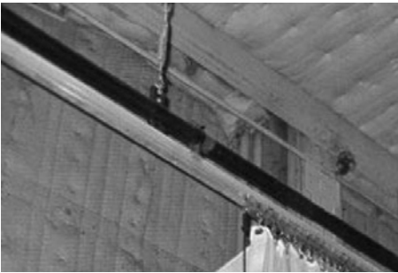
Figure 19.106 Day/night curtain on grid pipe system rail.
