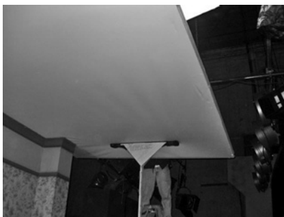
Figure 19.135 Lifting sticks used to move cloth-covered frame ceiling panels.
