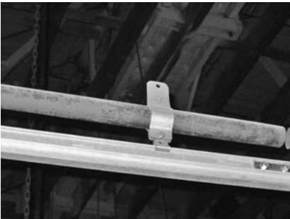
Figure 19.108 Grid pipe system rail.
