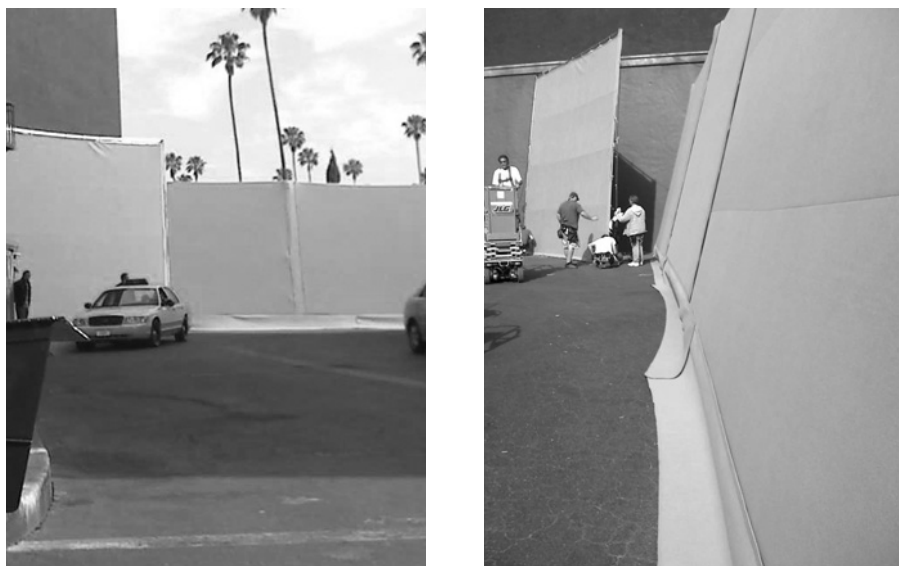
Figure 19.2 Notice the seams; we cover them with a Velcro-backed material.
