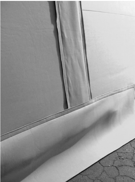
Figure 19.5 Seam cover strips.
