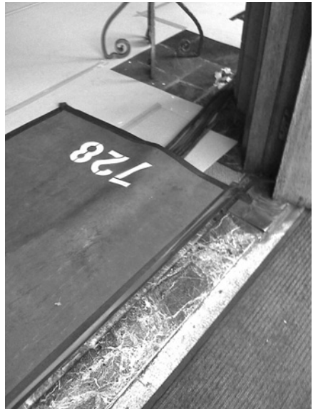
Figure 19.154 Rubber mat used to cover electric cables.
