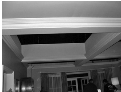
Figure 19.133 False ceiling removed.
