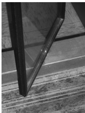
Figure 19.136 Pulling a set window.
