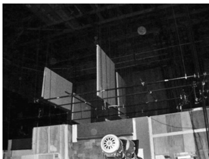
Figure 19.134 False ceiling hanging from perms.
