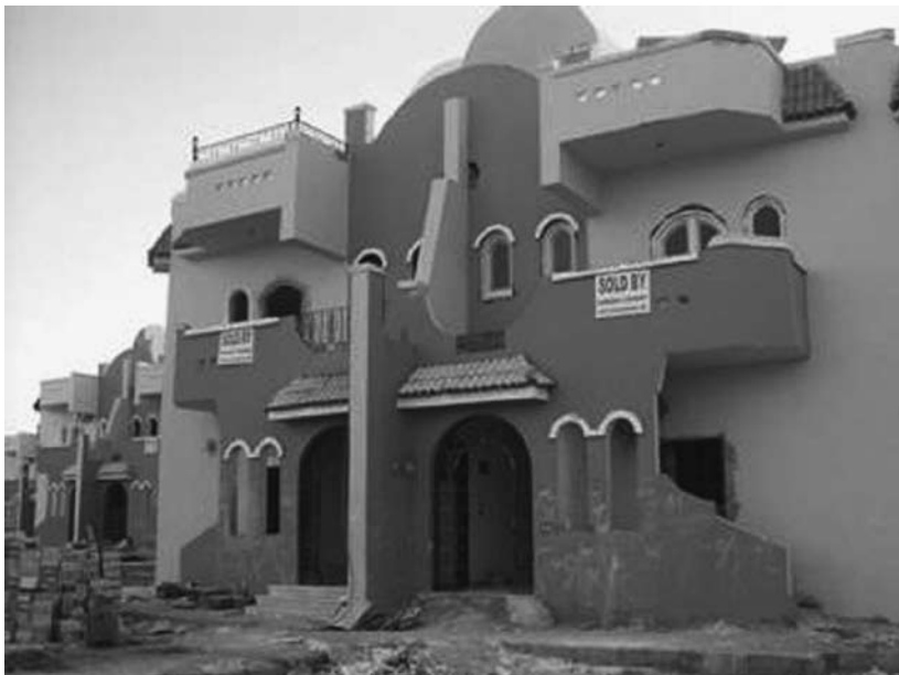
Figure 3.9 Second home under construction, Hurghada, Egypt
