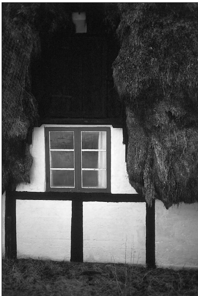
Figure 15.27: Thatching with eelgrass, Denmark.
