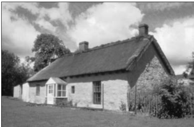
Figure 13.18: Recently renovated 200-year-old earth building in pisé construction in Perthshire. Source: Howard Liddell
