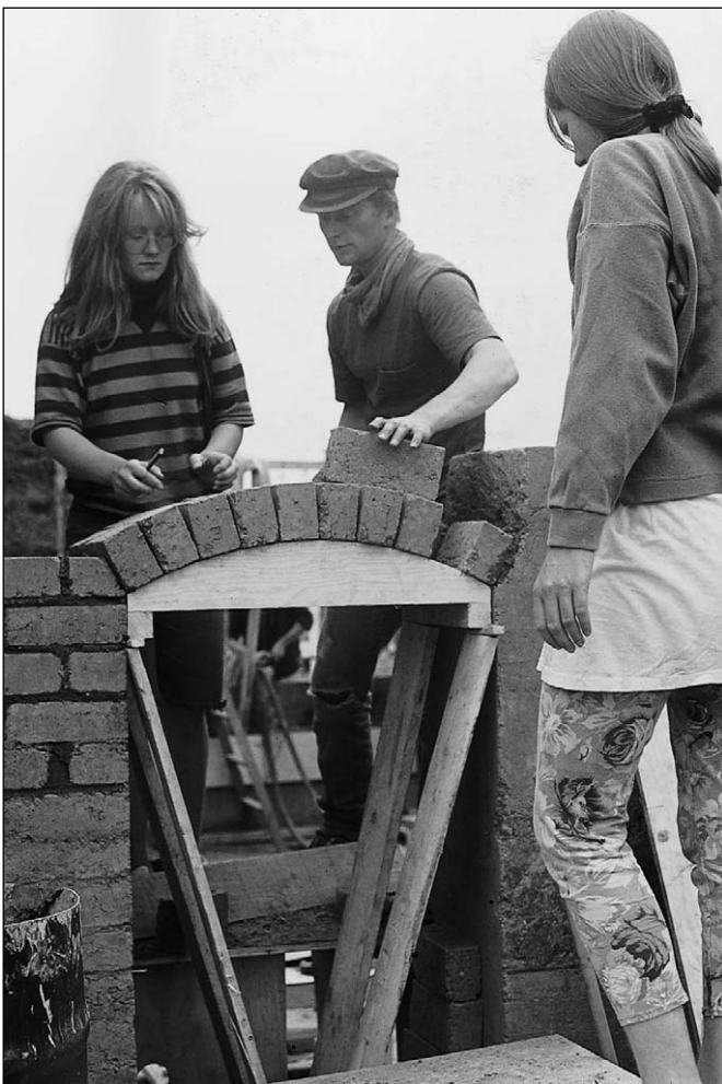
Figure 13.25: Building with earth blocks. Source: Gaia Lista 1991
