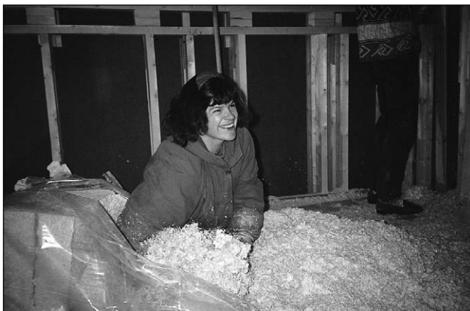
Figure 14.12: Thermal insulation made out of sawdust.
