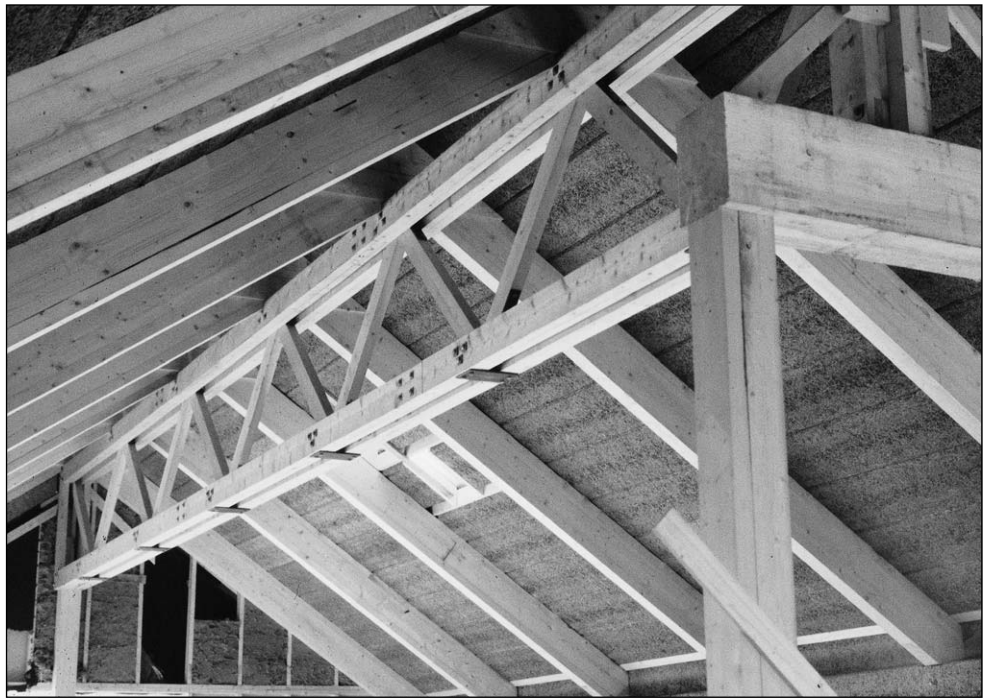
Figure 13.31: A lattice I-beam in a bakery. All joints are fixed by bolting; no glue is used. Source: Gaia Lista, 1990
