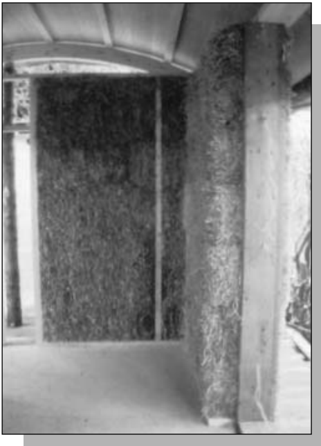
Figure 14.17: Straw bale building. Source: Howard Liddell
