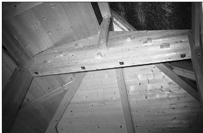
Figure 13.29: A roof joint bolted together, not glued, stiffened by dowels. Source: Gaia Lista, 1987
