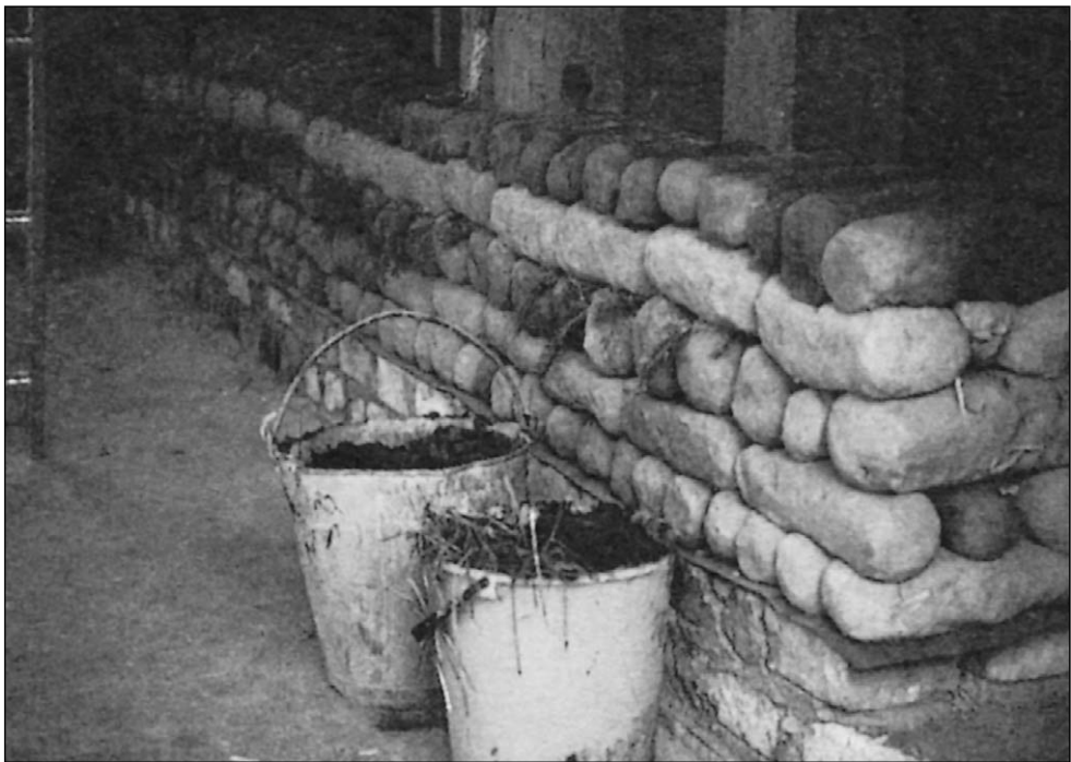
Figure 13.27: The earth loaf technique.
