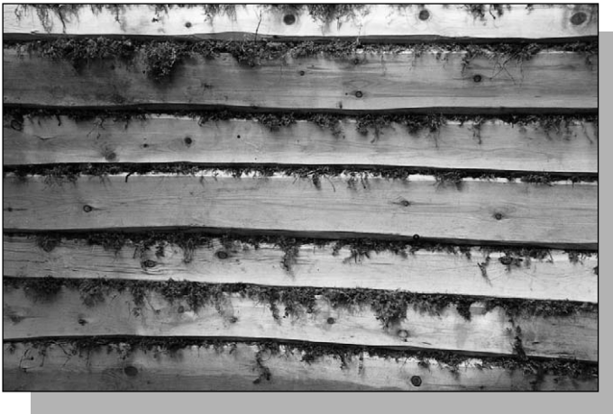
Figure 14.20: Log wall sealed with moss.
