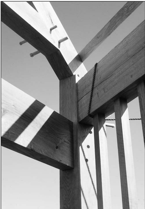
Figure 13.40: Traditional timber frame construction. Wooden plugs are used for fixing. Source: Gaia Lista, 1992
