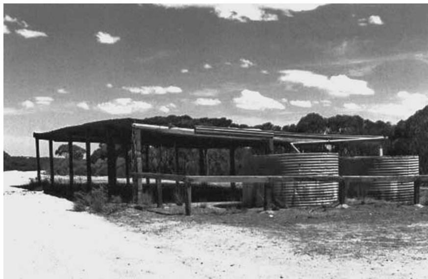
Illustration 7.3 Government Built Roadside Rainwater Catchment Tanks, Eyre Peninsula, South Australia
