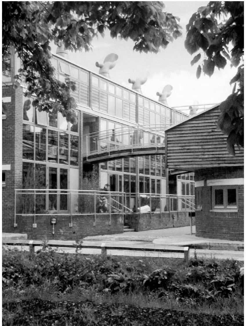
Figure 7.4 Southern elevation, BedZED housing development, South London
