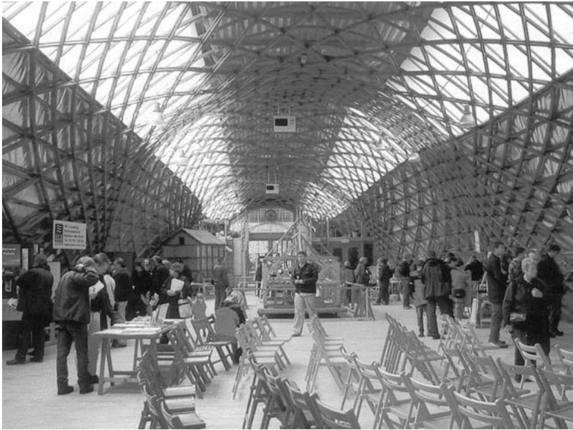
Figure 8.7 Interior of the Weald and Downland Conservation Centre (Edward Cullinan and Partners)
