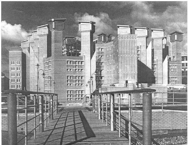
Figure 12.2 Coventry University library (courtesy of Marshalls plc)
