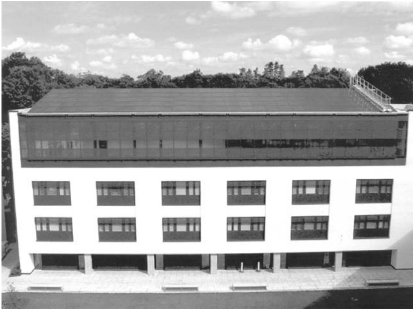
Figure 18.4 ZICER building south elevation with facade and roof PVs
