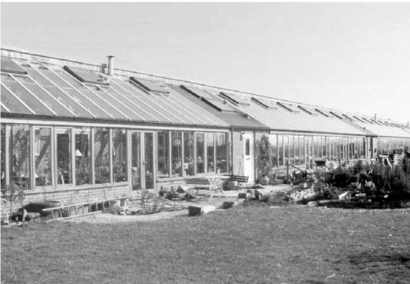
Figure 5.3 Passive solar houses, Hockerton Self-Sufficient Housing Project 1998
