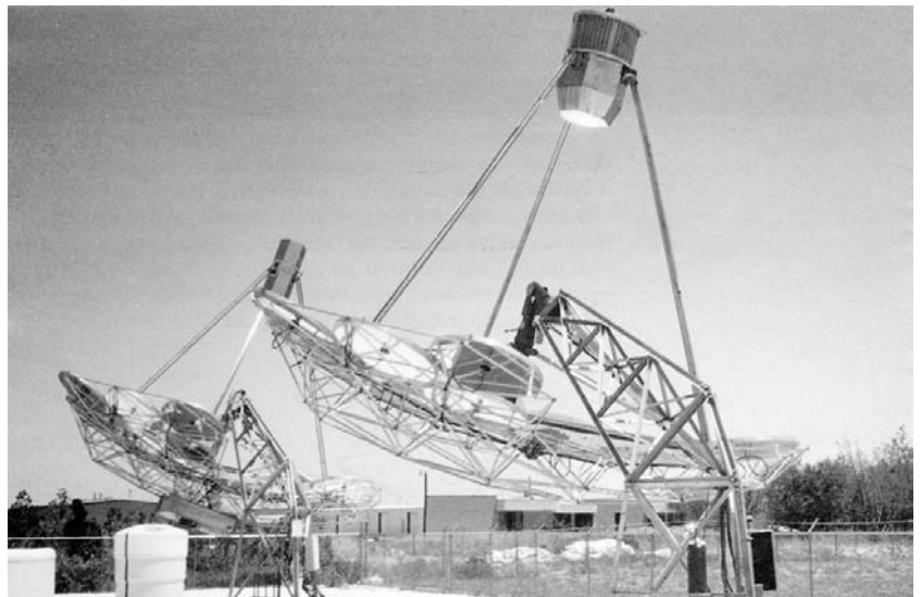
Figure 4.2 Solar concentrator, Abilene, Texas (courtesy of CADDET)
