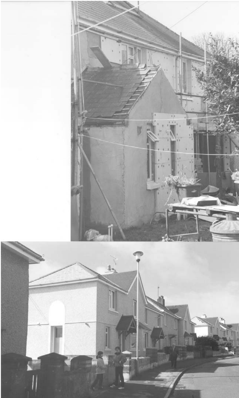
Figure 10.1 Social housing with cladding over solid wall construction, Penzance
