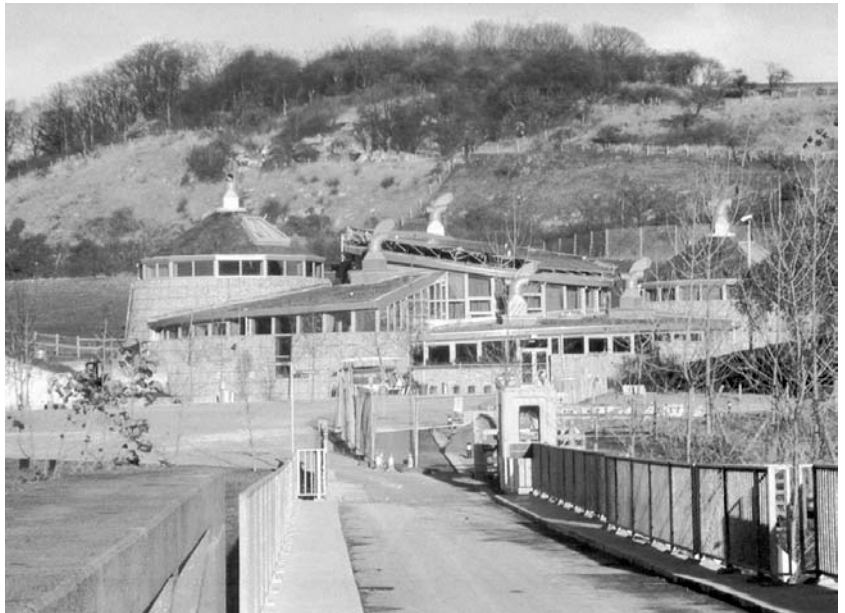
Figure 17.1 Conference Centre, Earth Centre, under construction and completed
