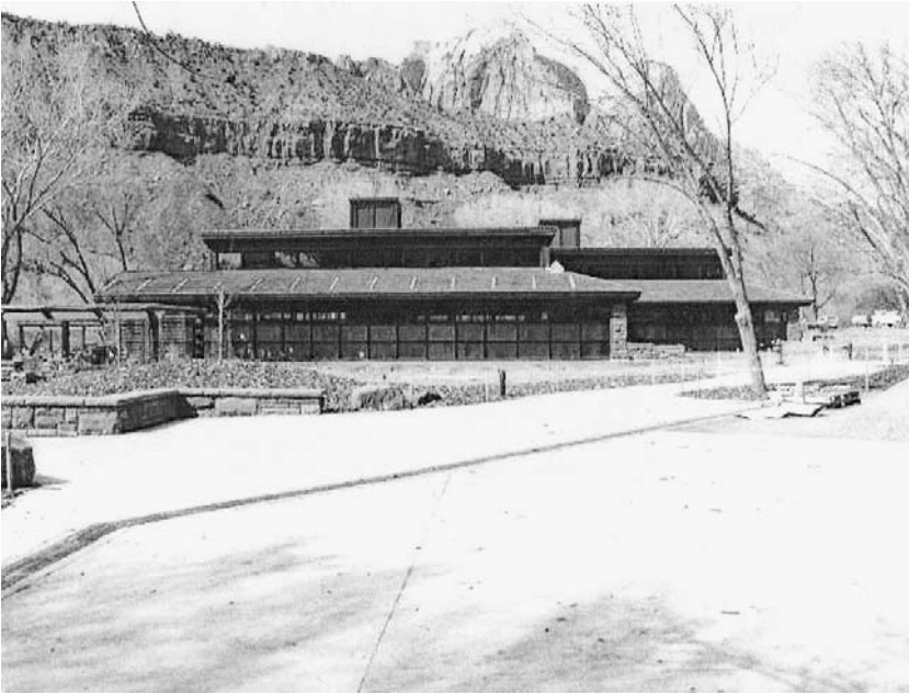
Figure 20.1 Zion National Park Visitor Center showing cooling towers and Trombe wall
