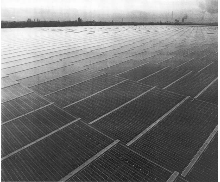
Figure 13.5 PV roof over the Mont Cenis complex, Herne Sodingen, Germany
