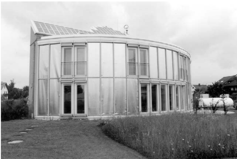
Figure 5.6 Freiburg Solar House showing Trombe walls with blinds in operation. Note the hydrogen storage tank on the right
