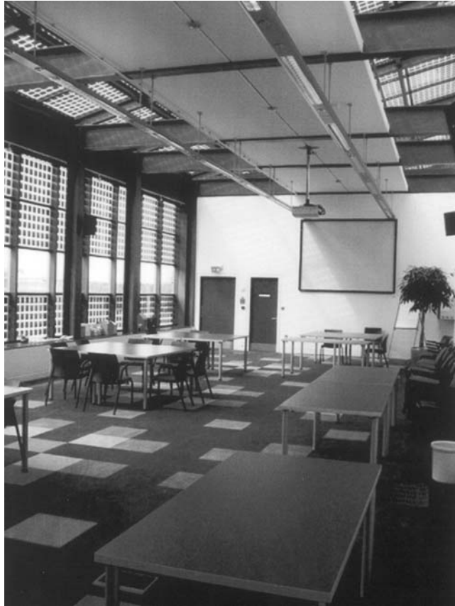
Figure 18.5 ZICER building Seminar Room with facade and roof PVs and thermal mass suspended ceiling panels
