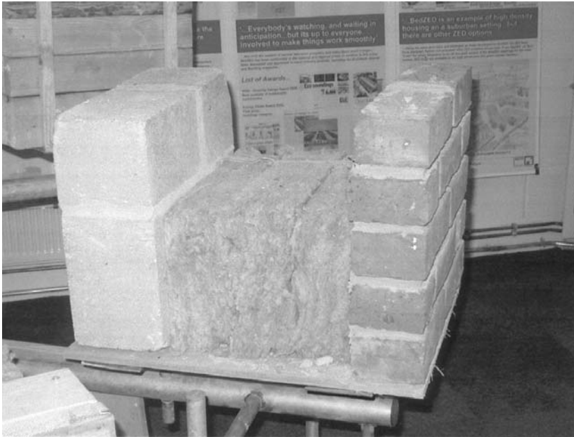
Figure 18.9 Masonry wall construction
